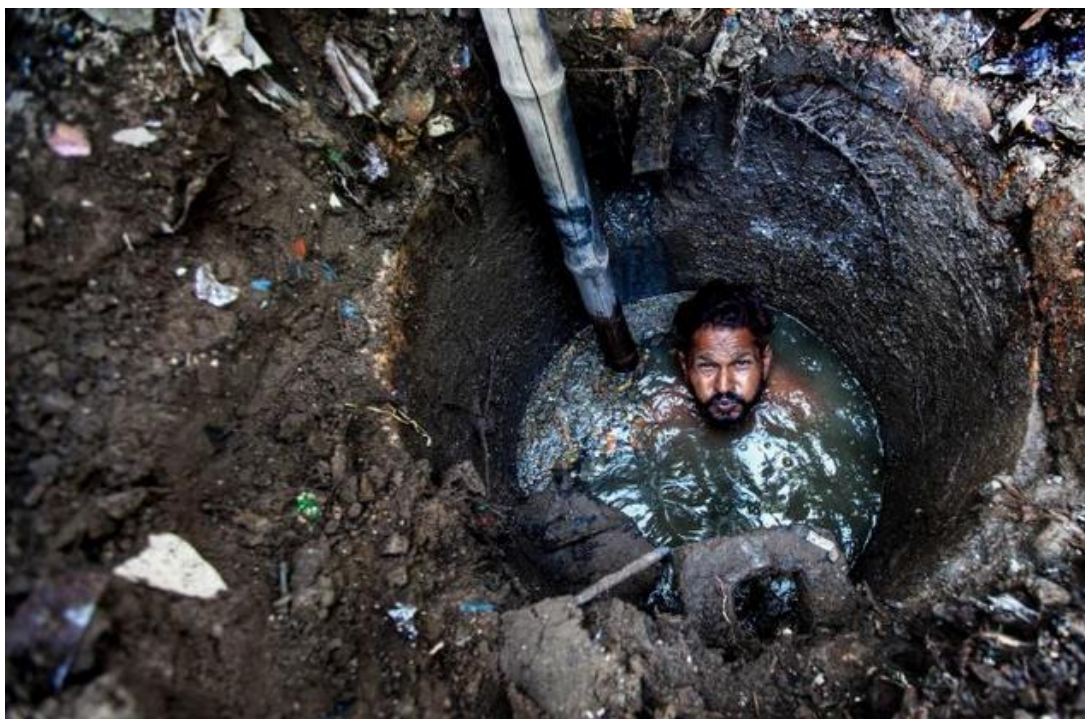
The manual scavenger has to enter the drains barefoot and without a mask. He ends up inhaling toxic gas and swallowing dirty water, but now considers these as unavoidable occupational hazards. | Photo Courtesy: Vijay Pandey/TwoCircles.net
