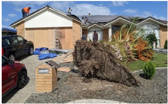
Tornado damaged house in Auckland. Photo Credit: RNZ
