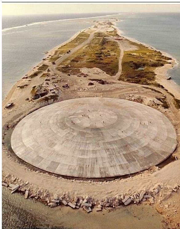
Runit Dome (or Cactus Dome), Runit Island, Enewetak Atoll. Aerial view. In 1977-1980 the crater created by the Cactus shot of Operation Hardtack I was used as a burial pit to inter 84,000 cubic meters of radioactive soil scraped from the various contaminated Enewetak Atoll islands. The Runit Dome was built to cover the material..資料：US Defense Special Weapons Agency, Public
